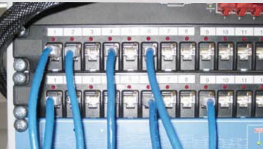
Guided changes: LEDs at the patch panels show which cables are to be plugged in elsewhere.
