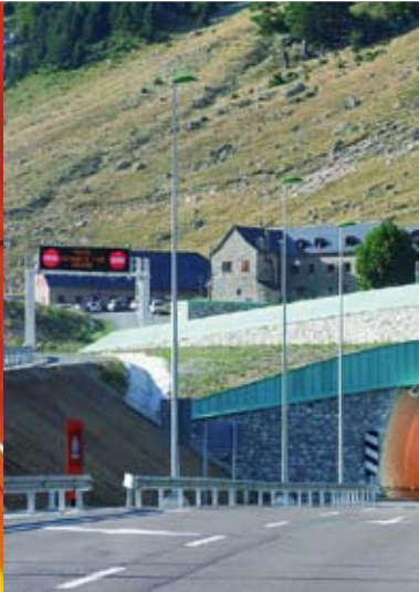
Vielha Tunnel | Spain
