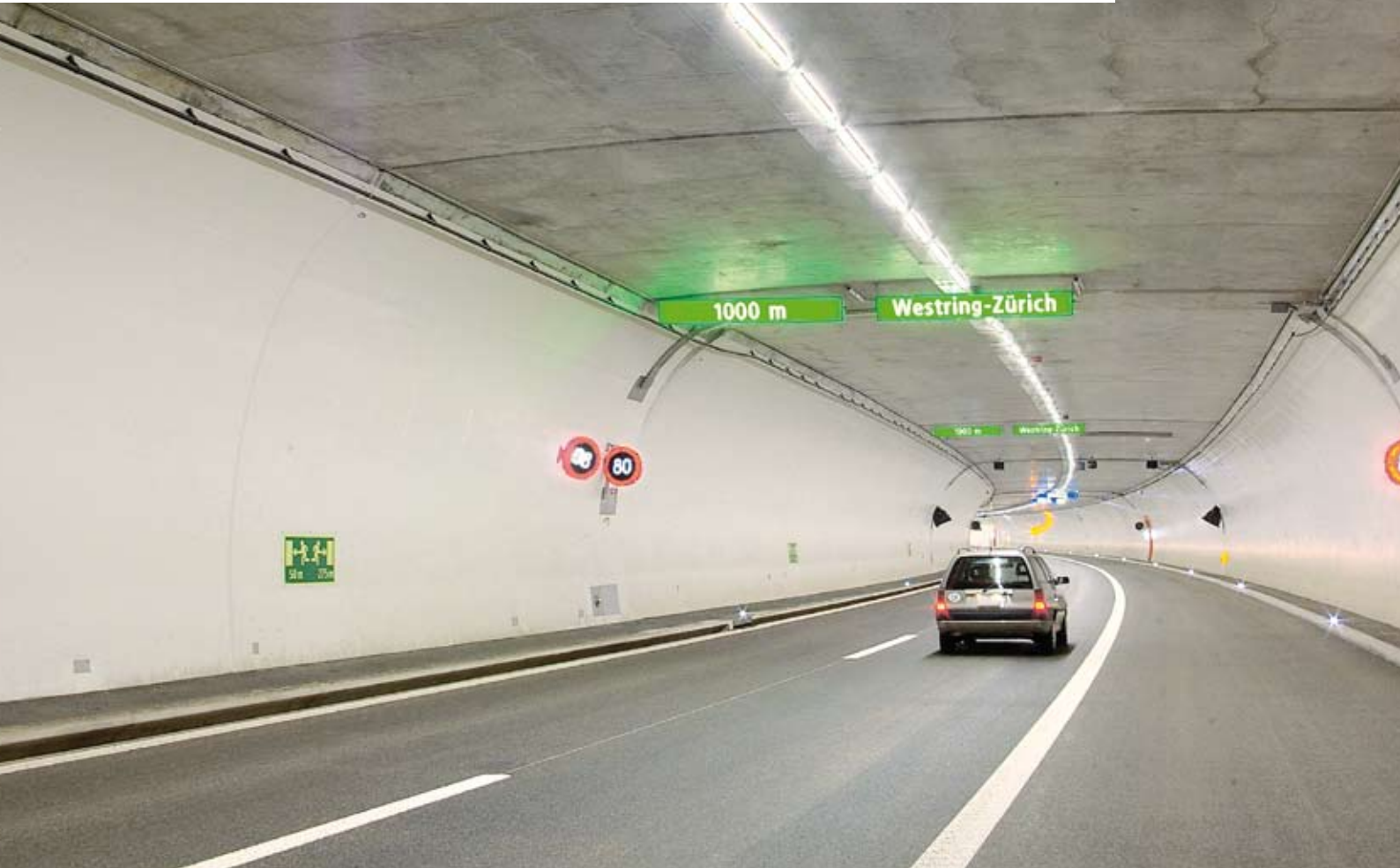
Uetliberg Tunnel | Switzerland
